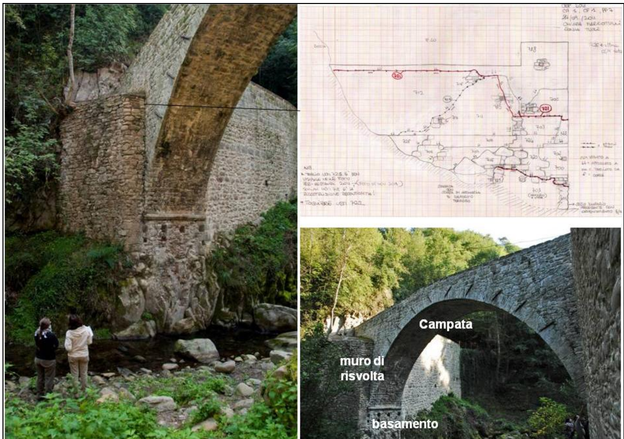
Fig. 19. Stratigraphic readings at the Bridge of Sant'Angelo in Cetica (elab. Chiara Marcotulli)
