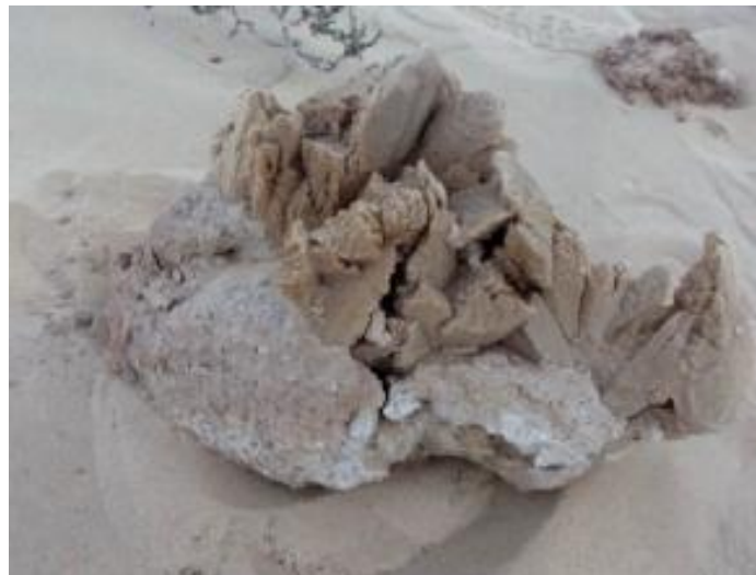
Figure 6. Stone and mortar of a wall of an old rural house in the Souf [5].
