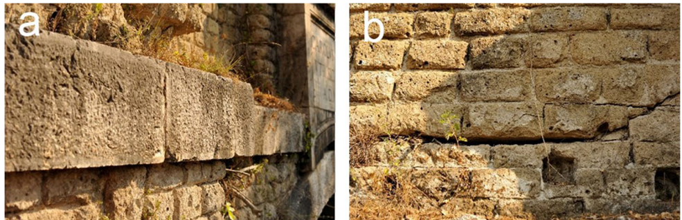
Fig. 4 The main materials of the Bridge: a the local limestone with the presence of a disintegration phenomenon and a superficial patina; b the yellow tuff, and the clear lesion on the South elevation
