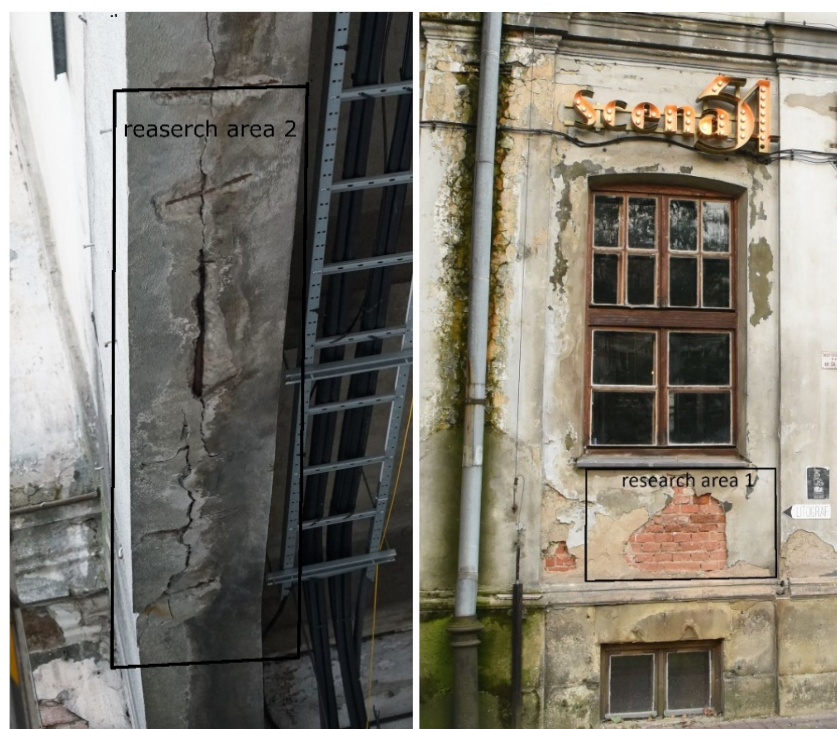
Figure 3. The research objects (1-wall with damaged plaster on the left, 2-concrete element with the cracks on the right).
