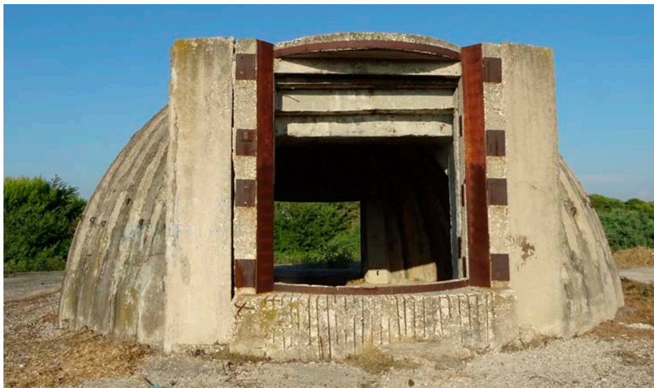
Figure III-3.10 Two views of the monumental bunkers located on the plain of Zhukë.
