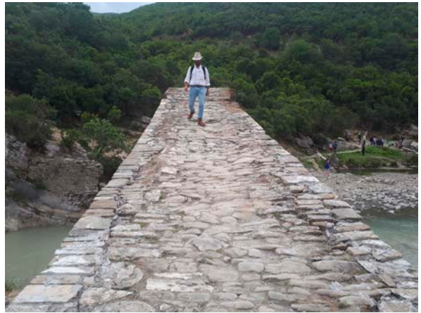
Figure I-5.1.4 – The roadway of the bridge.
