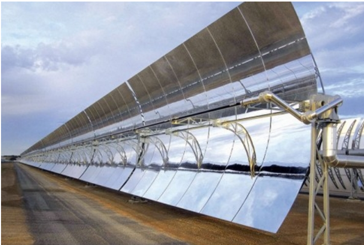
Figure 1.5: Example of big PTCs: Noor I CSP in Morocco.
