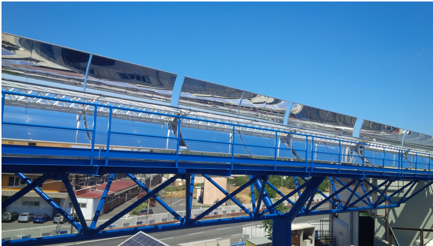
Figure 1.9: PTC installation in Catania realized by the University of Florence.
