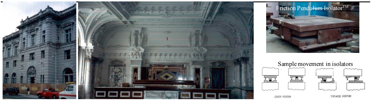
Fig 8. Base isolated monumental building of Court of Appeals – San Francisco, CA – with multiple artifacts.
