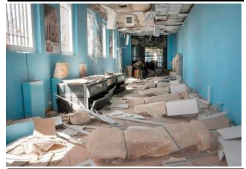
Fig. 6. Fallen statues and ceilings, damaged artifacts, due to external explosions (similar to earthquakes) in Palmyra, Syria
