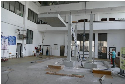
Slab placing on columns' top
