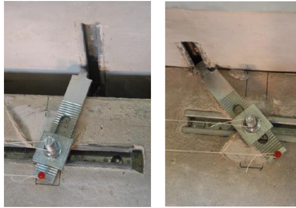
Figure 3-75: Hammer-head strap connection tested at UNI-LJ (Isaković et al., 2013)
