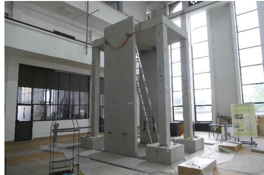
Complete structure with vertical panels assembled
