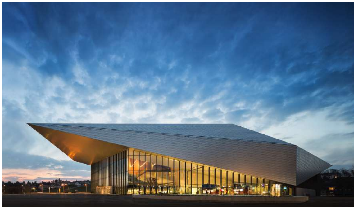
Figura 5. Vista dello Swiss Tech Convection Centre [Foto: ©Fernando Guerra].
