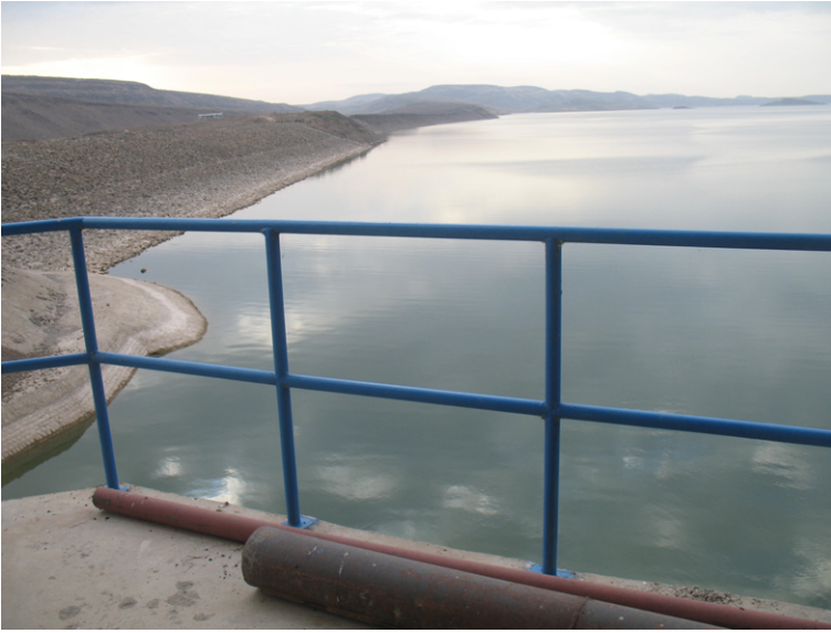
Fig. 2. Reservoir view seen from the intake tower.
