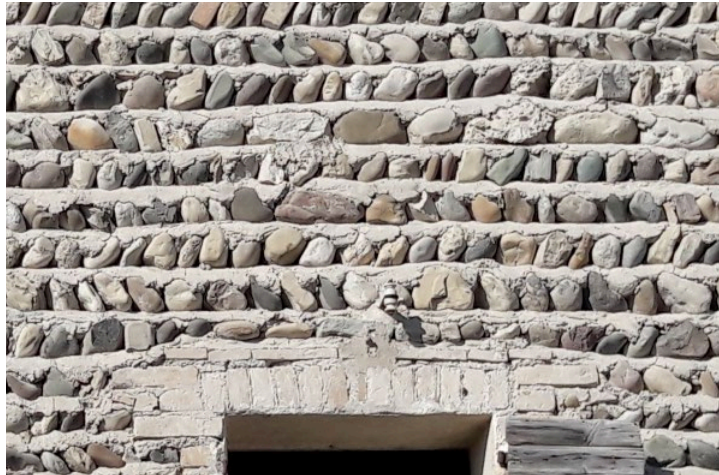
Fig. 3 – Wall made by Piave stones. Source: R. Z., 2018.
