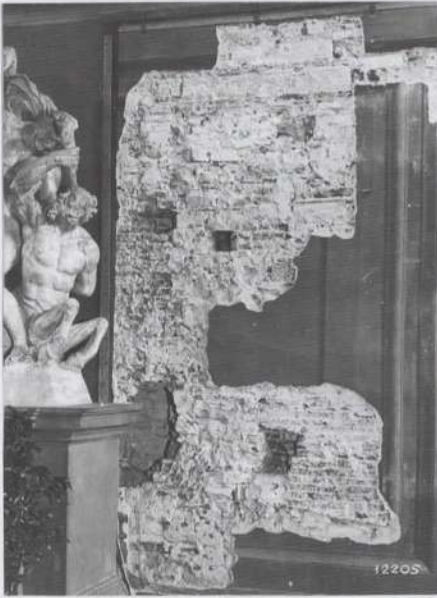
Figure 4. Detail of the masonry emergencies and the existing infilled openings included in Micheli's drawing (Fototeca Musei Comunali, raccoglitore 8 cod 81043).
