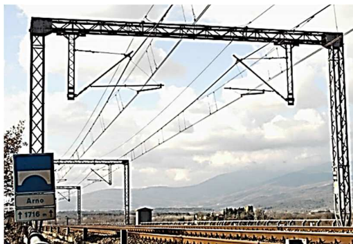
402 Figure 15: Catenary of the Firenze-Roma “Direttissima” High-speed Line.
