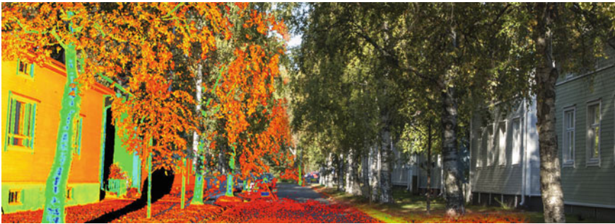
Fig. 6 The study case of the historic district of Raksila in Oulu, Finland. Laser scanning survey, analysis and documentation of the street facades with census activity of the architecture and its environment. Analysis and results included in the report Özlem Özer-Kemppainen (edited by Özer-Kemppainen 2017)
