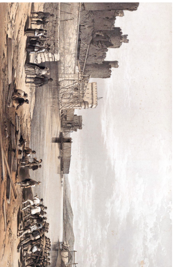
Figure 15 George Hawkins, Lithograph showing the second wrought-iron box girder tube of Robert Stephenson's tubular railway bridge at Conway being floated into position (September 1848), 300 × 465 mm (image), 370 × 547 mm (paper). Impression digitized by National Library of Wales. © Wikimedia Commons
