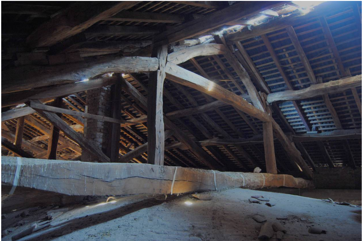
Figure 6: Truss number 3 (photograph by the author).
