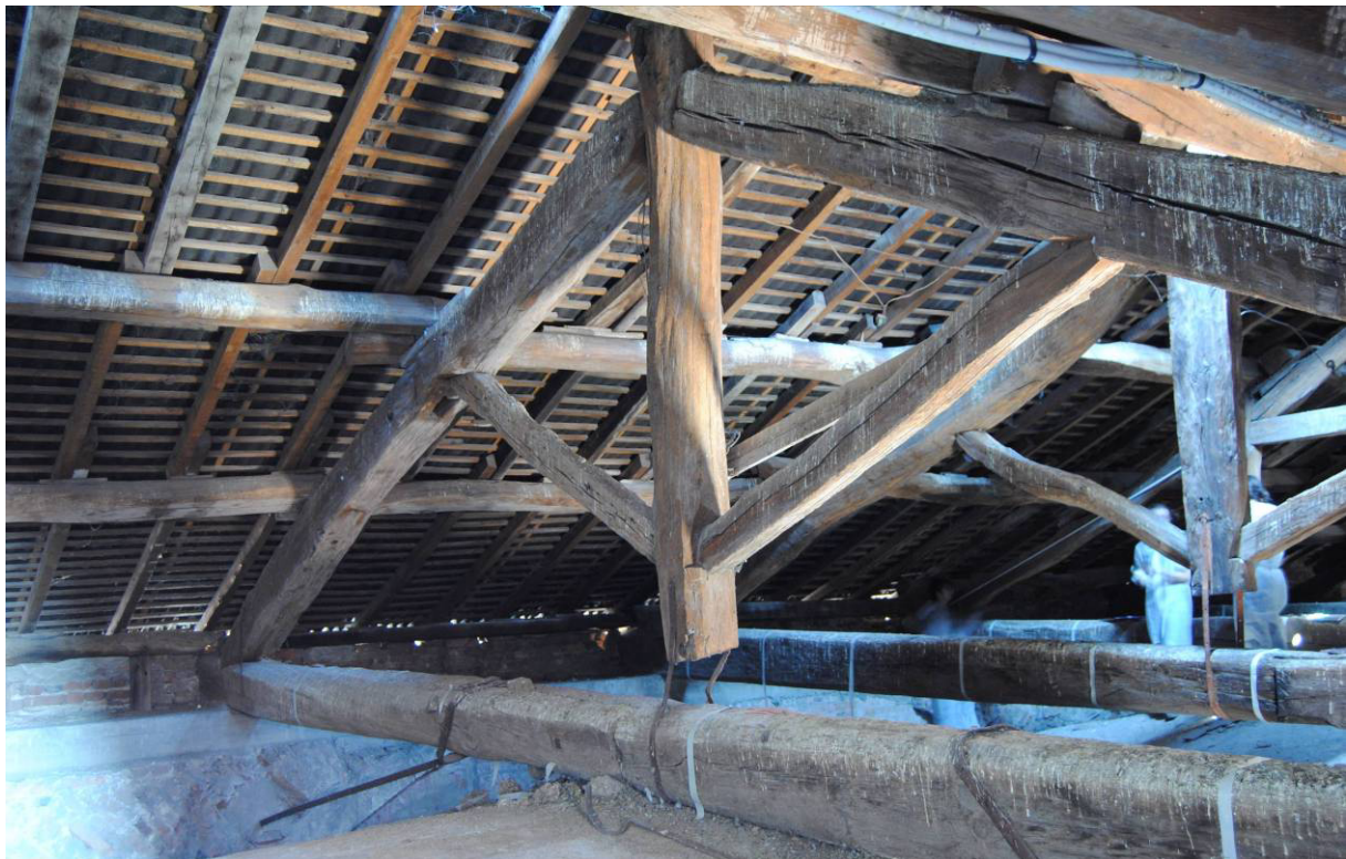
Figure 9: Truss number 1 (photograph by the author).
