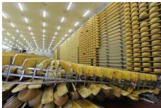
Figure 2-2: Collapse of some racks with parmesan wheels, placed inside a warehouse in Emilia Romagna, after the “Emilia earthquake” took place on the 20 th of May in 2012.
