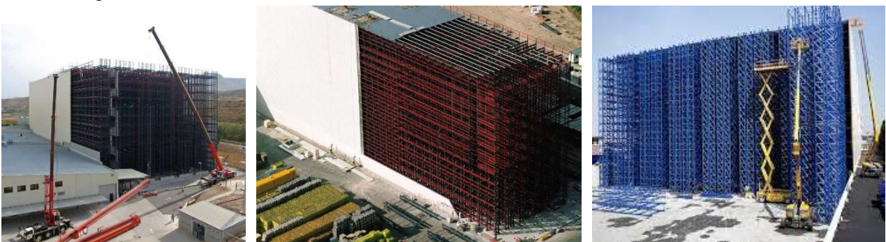
Figure 2-4: Some examples of existing ARSWs ( https://mecalux.it/ for the two figures, and https://sacmaspa.it/ for the last one).
