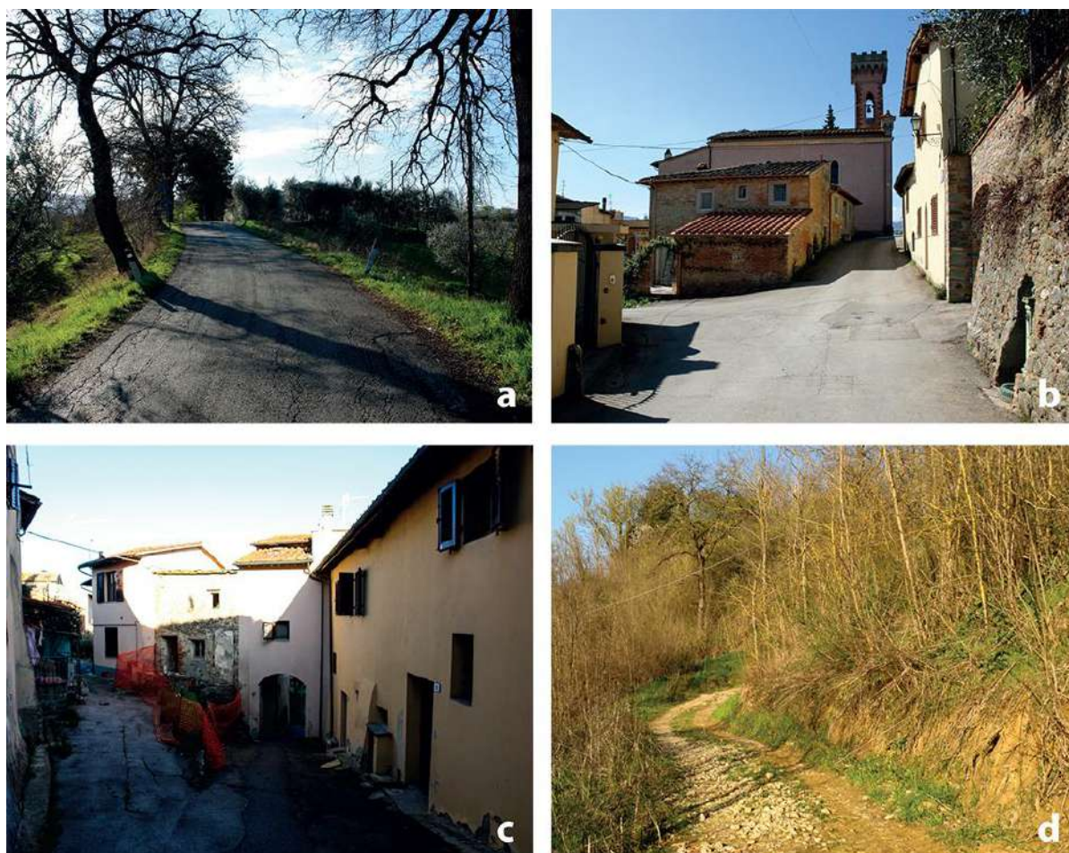
Figure 23 – In Ricasoli village the main constructive characteristics of infrastructures are summarized through four different types, previously described. In the figure, a) Type A, b) Type B, c) Type C and d) Type D are reported.
