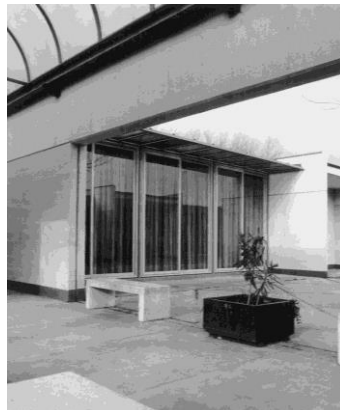
Figure 2.8 Window of a classroom for connection with the garden in Ai Saleggi kindergarten – Reference: http://www.studiovacchini.ch/opere/10
