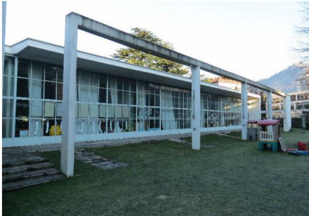
Figure 2.5 Glass facade of classrooms – Reference: http://www.maarc.it/opera/asilo-infantile-antonio-santelia
