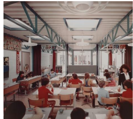
Figure 2.9 Skylight of a classroom – Reference: http://www.studiovacchini.ch/opere/10
