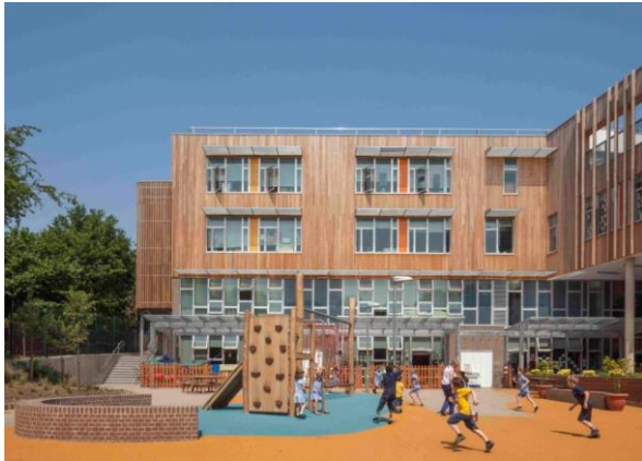
Figure 2.27 Primary school Ashmount internal courtyard view
