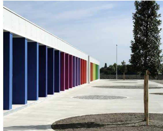
Figure 3.29 One of main facade of Zugliano school – Reference: www.theplan.it
