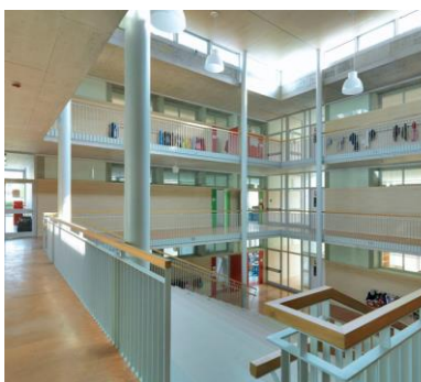
Figure 2.36 Internal view of Romarzollo elementary school atrium
