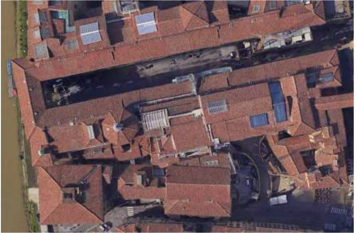
Fig. 5. The roofs of the Uffizi complex.
