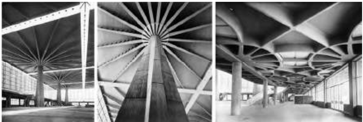
Fig. 5. The palace of Labor interior (TSLF), Fig. 6. Detail of the pillar (TSLF) and Fig. 7. Detail of the ribbed ceiling of the gallery (TSLF).
