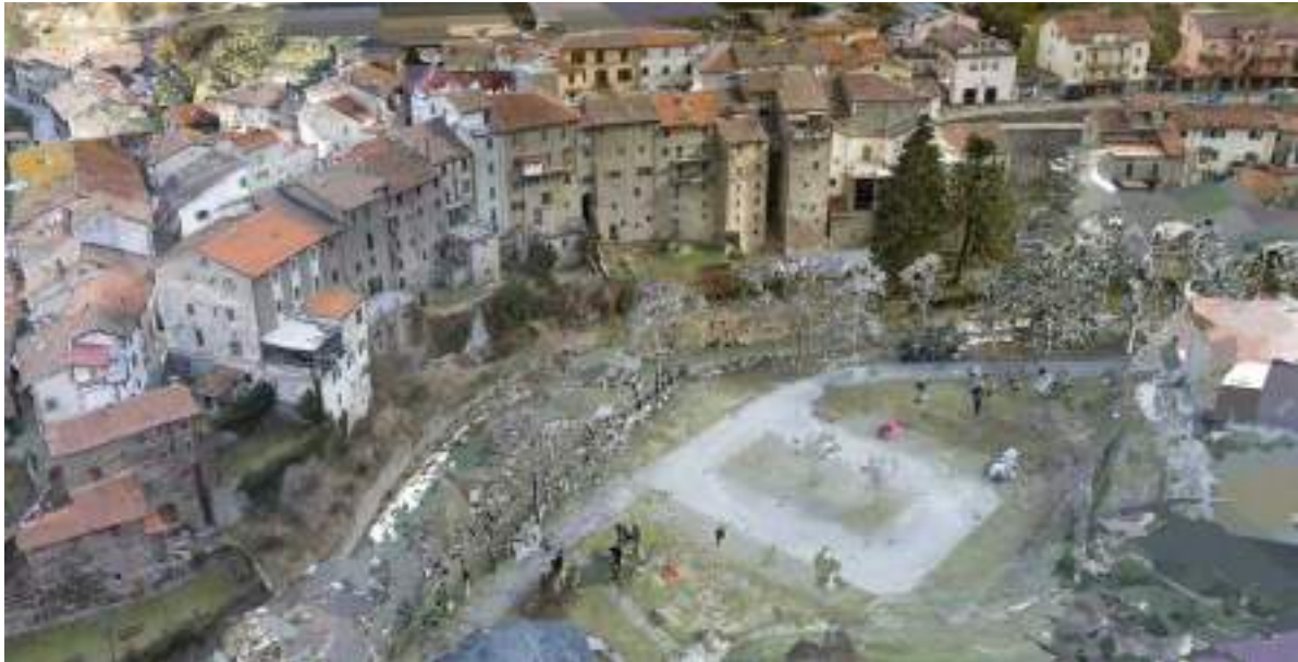
Fig. 2. Texture model processed in RealityCapture - UAV drone photogrammetry.
