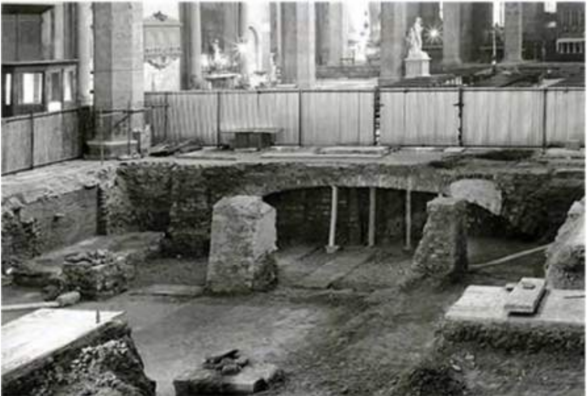
Fig. 8. One of the 1967 photographs of the foundations of the tramezzo , uncovered during archeological excavations.
