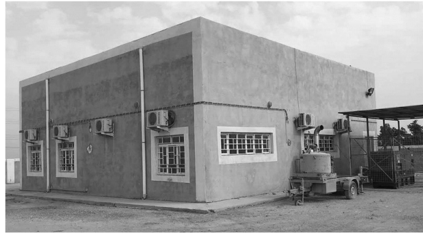
Figure 1. Dairy factory building, south-west side.
