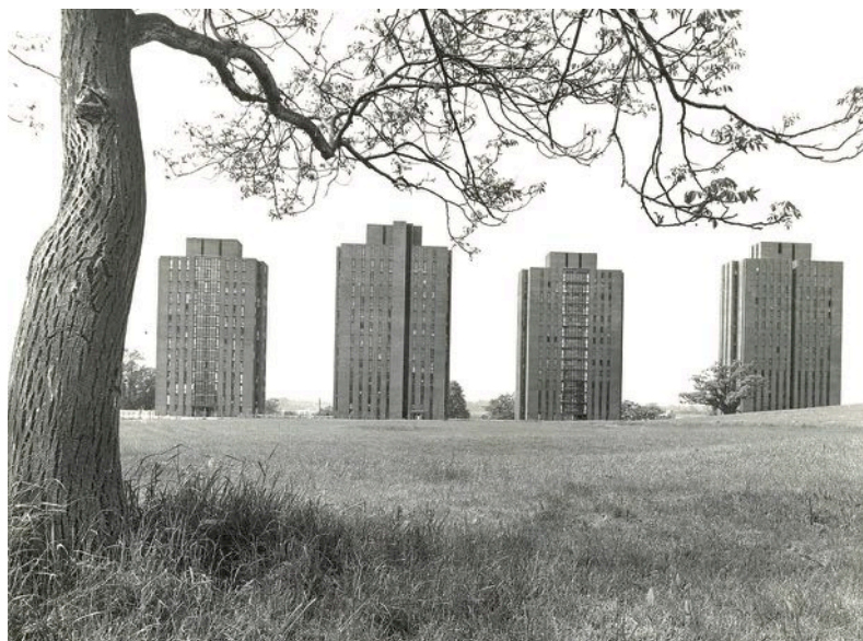
Figure 12.3 The monumental residential towers at Essex, on the skyline and contrasting with the trees in the parkland
