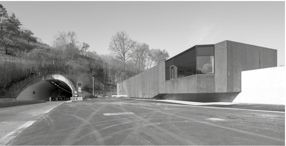
Bundesbau Baden-Württemberg, Tunnel Service Facilities, view from the federal highway, Waldkirch, 2019.
