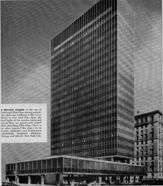
**A BRILLIANT EXAMPLE** of the use of Pittsburgh Plate Glass among present-day glass-clad buildings is the Lever House in New York City. Here, the floor lights of the massive tower and second floor are glazed with Sobex® Heat-Absorbing Plate Glass. There is no other material like glass – in its beauty, modernity, and architectural adaptability. Architects: Skidmore, Owings and Merrill, New York City.
