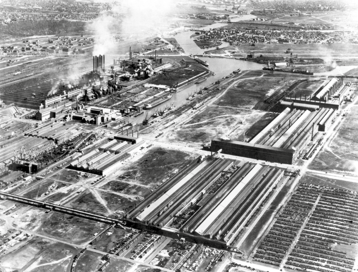
Albert Kahn, Inc., Ford Motor Company, River Rouge Plant, Dearborn, MI, 1938.
