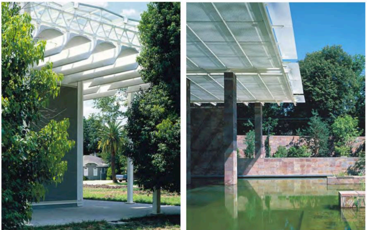
Fig. 11-12. On the right, the layered roof structure of the Fondation Beyeler in Basel as a reinterpretation of the Menil Collection's one, on the left (Renzo Piano Foundation, Genoa).
