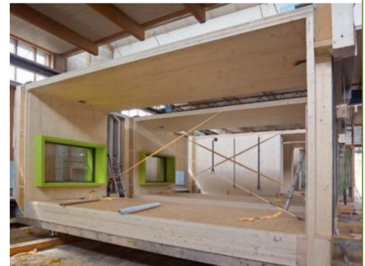
Image 02 – Modular units can be off-site finished with exterior cladding, internal finishes and doors and windows
