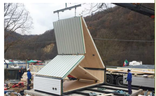
Image 03 – In order to optimize transport, MADI Home has patented a pop-up residential modular unit built with CLT technology Credits: MADI Home
