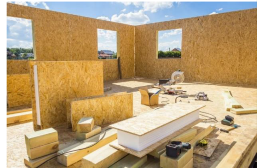
Image 01 – SIP Panels being installed on site for further integration
