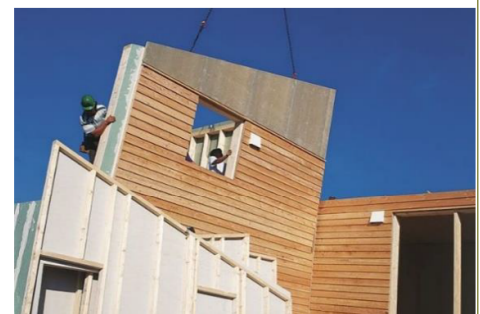
Image 03 – Wood framed panels during installation phases
