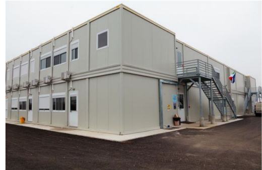
Image 01 – Portable modular units employed for a post-earthquake school (Malpighi School in Mirandola, Italy)
