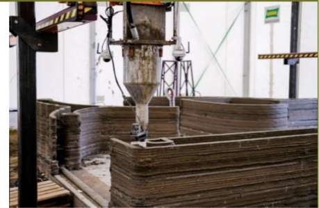
Image 01 – 3D printing machine used for residential building project Credits: COBOD
