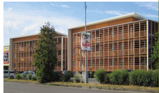
Image 01 – Wooden modular units employed for Temporary Social Housing (Florence, IT - 2013), the first building in Italy delivered with wooden units
