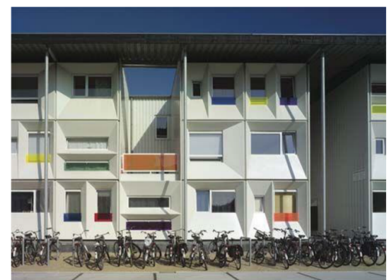
Image 03 – Common use in architecture for modular shipping containers is student housing, because of their space repeatability. In the picture, Qubic Student Housing in Amsterdam (Netherlands) by Studionedots
