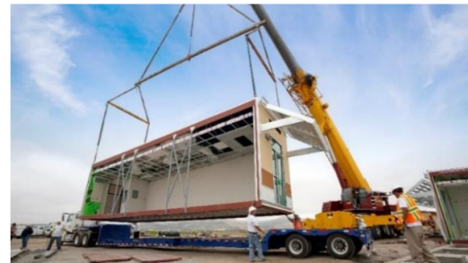
Image 02 – Installing sequences of steel modular units Credits: American Modular Systems (AMS)
