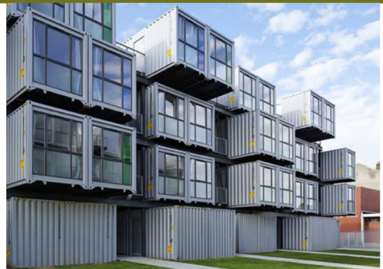
Image 01 – Shipping containers used in Cité A Docks in Le Havre, France
