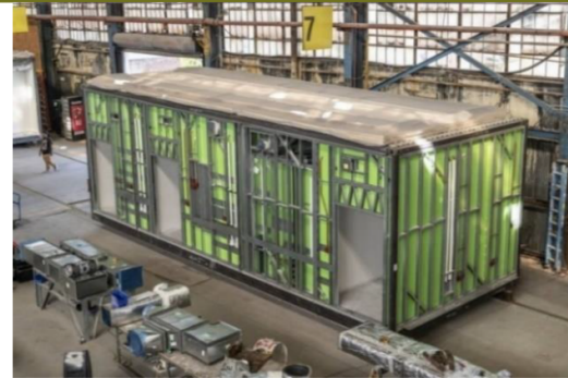
Image 01 – Modular units are off-site manufactured following streamline sequences of assembly Credits: American Modular Systems (AMS)
