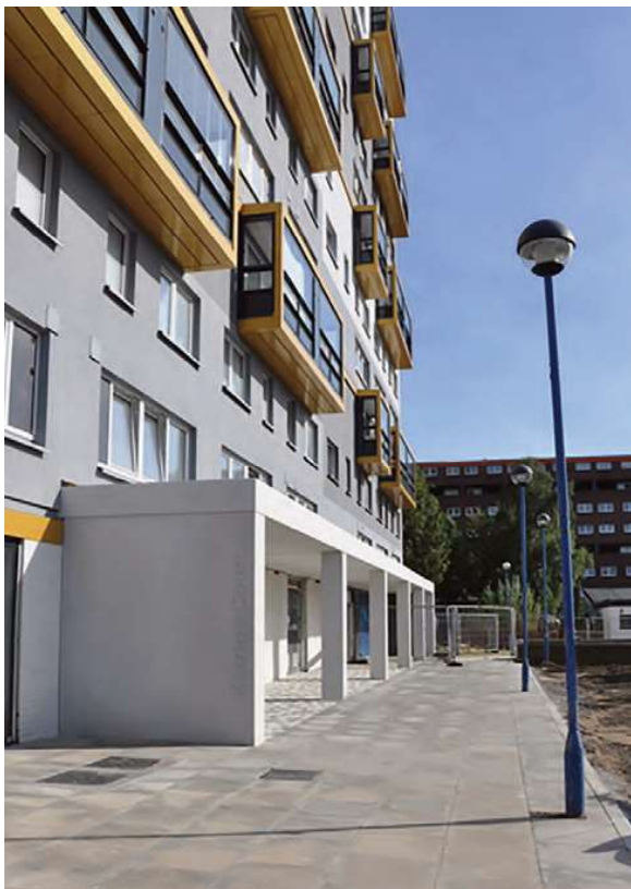
Fig. 4 | Woodside Multi Storey Flats after the retrofit, by Collective Architecture, Glasgow (credit: Collective Architecture, 2019).
