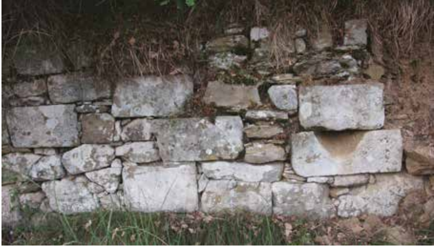
Fig. 4 and 4a The terracing in the locality of San Giovanni alle Balze in which they are evident materials of recovery from buildings of greater relief in fig. 4 is visible also the arc (inverted) of a single-hole.
