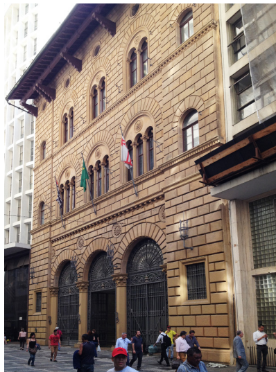
Fig. 9. Photo of the Banco Santander in Rua Quinze de Novembro, with the peculiar facade in 'Florentine' style (photo by the authors); Detail of the facade of the Hotel Jaraguá, 1948, by F. Heep and M. Juliano.
