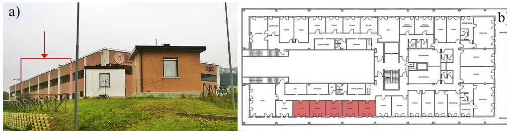
Fig. 1. (a) Picture and (b) plan view of the monitored institutional building in Perugia, Italy.
