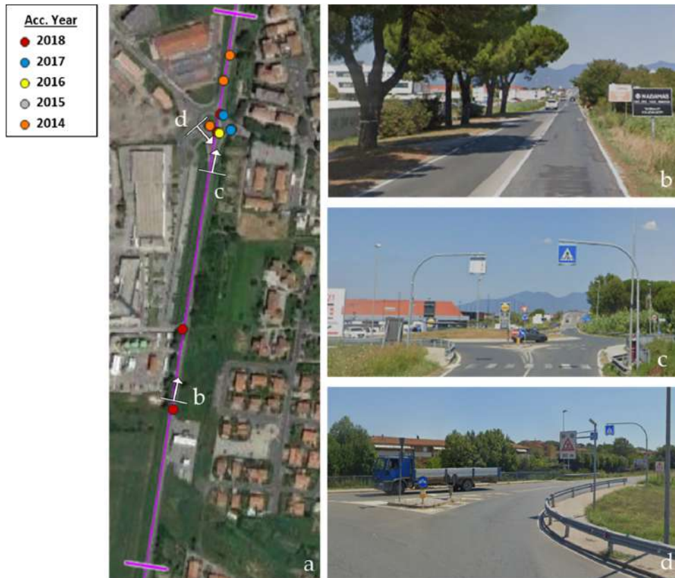
Figure 11. SR206_032_1 HS with accidents' location on a satellite image (a) and two pictures of the HS in the northbound direction (b,c), and one in the southbound direction, exiting the roundabout (d).
