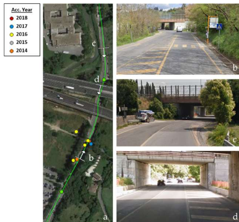
Figure 8. SR2_291_0 HS with accidents' locations on a satellite image (a) and two pictures of the HS in the northbound direction (b) and one in the southbound direction (c,d).
