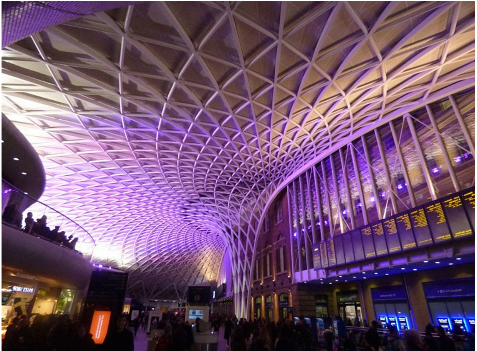
Figure 9. King's Cross Station, London - 2012
