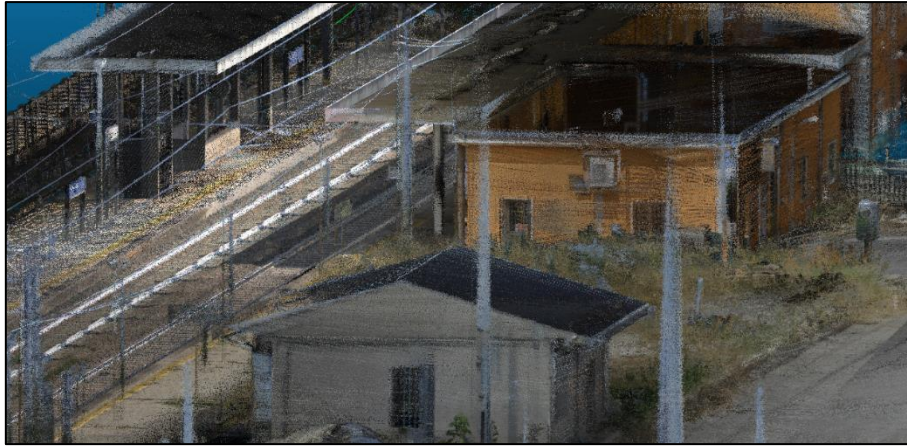
Figure 31 - compound train and backpack LIDAR data in the station zone
