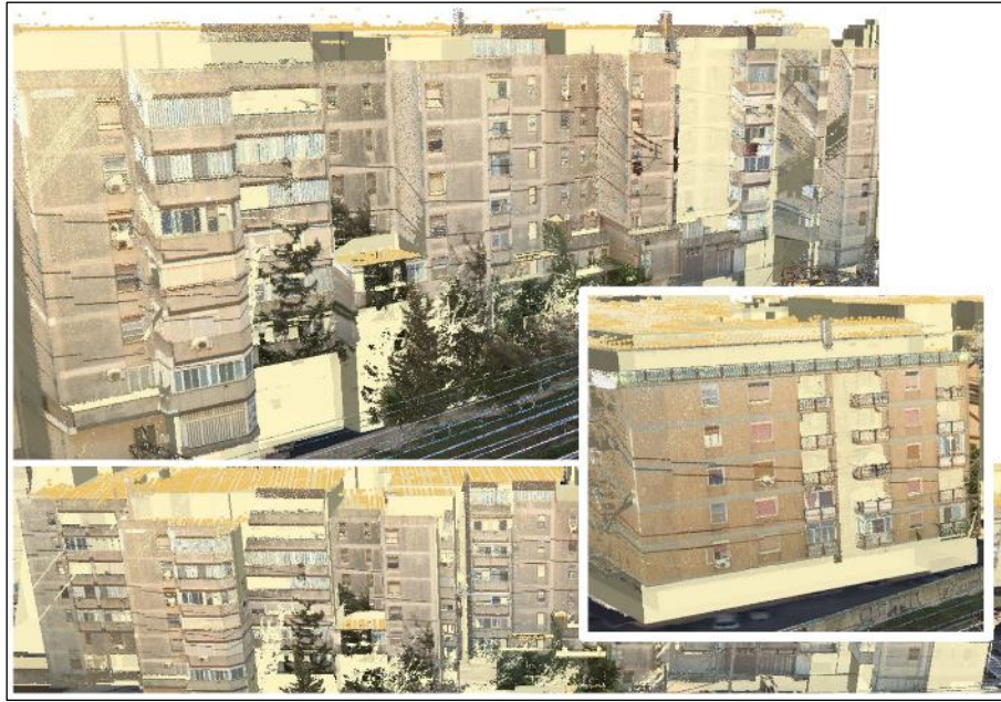
Figure 66 - Point clouds of façades from telemetry survey of the case study (chapter 5).
