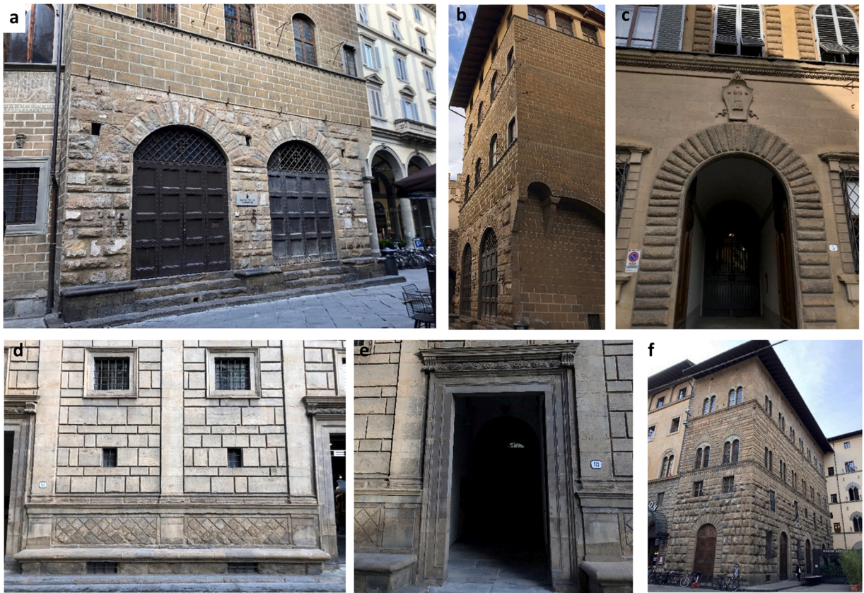
Fig. 3. Some examples of the use of Pietraforte for architectural details. a, b. Palazzo Giandonati (base and arches), c. Palazzo Torrigiani (frame), e, f) Palazzo Rucellai (frame and base); g) Strozzino (string courses, vestment).
