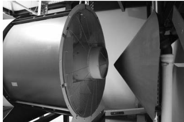
(c) Close-up of the motor fan
