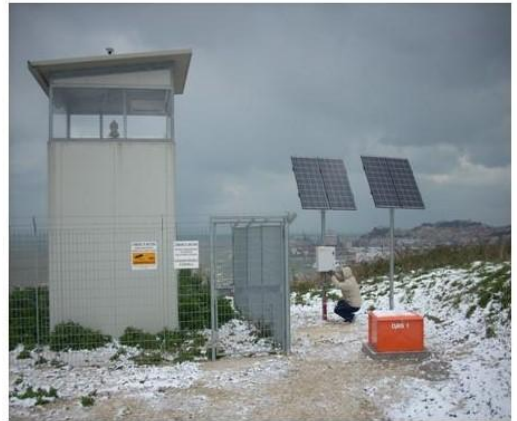
Figura C.27 - Main station Grotte
