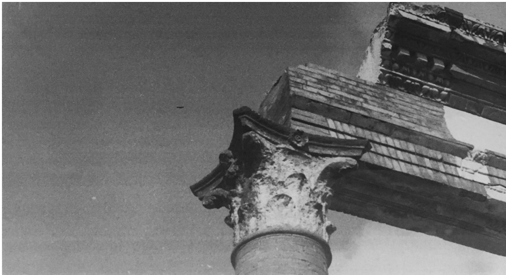
↑ Focus of a column in the Forum of Pompeii: Corinthian capital and its entablature. (Analogic photo by the author).
