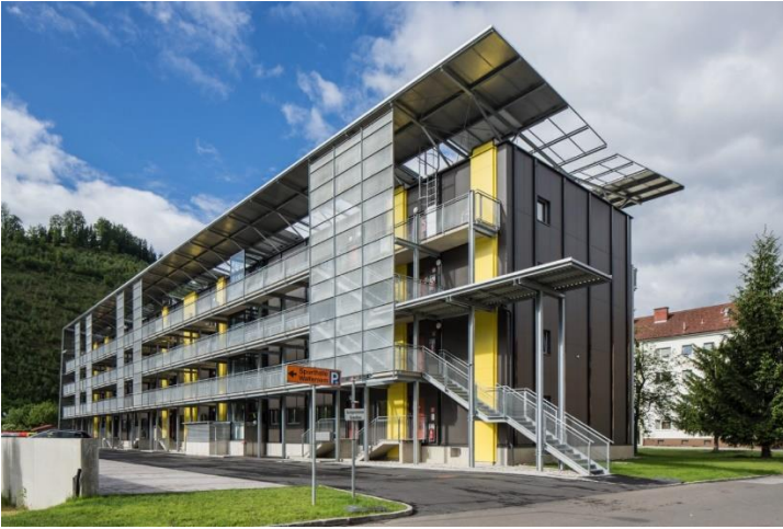
Fig. 04 | A building of Kapfenberg District after the deep renovation. Photo by: Walter Luttenberger
