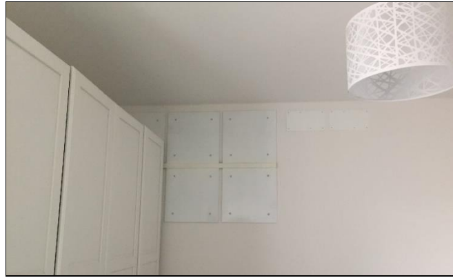
Fig. 3 - Layout of the flux tiles in one bedroom. In the white boxes on the right, cables are collected and sent to Data Acquisition Unit.
