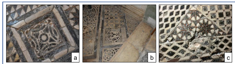
Figure 4. Fracture (a,b), loss of material (a–c), discolouration (b), differential erosion (a,c), lacunae (c).
