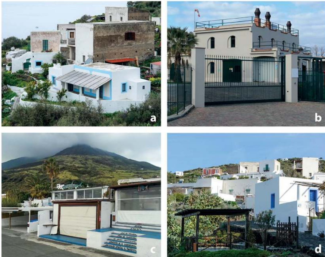
Fig. 4. The main constructive characteristics of buildings on Stromboli Island, summarised through four different types. In the figure, a) Type A, b) Type B, c) Type C, and d) Type D are reported.
