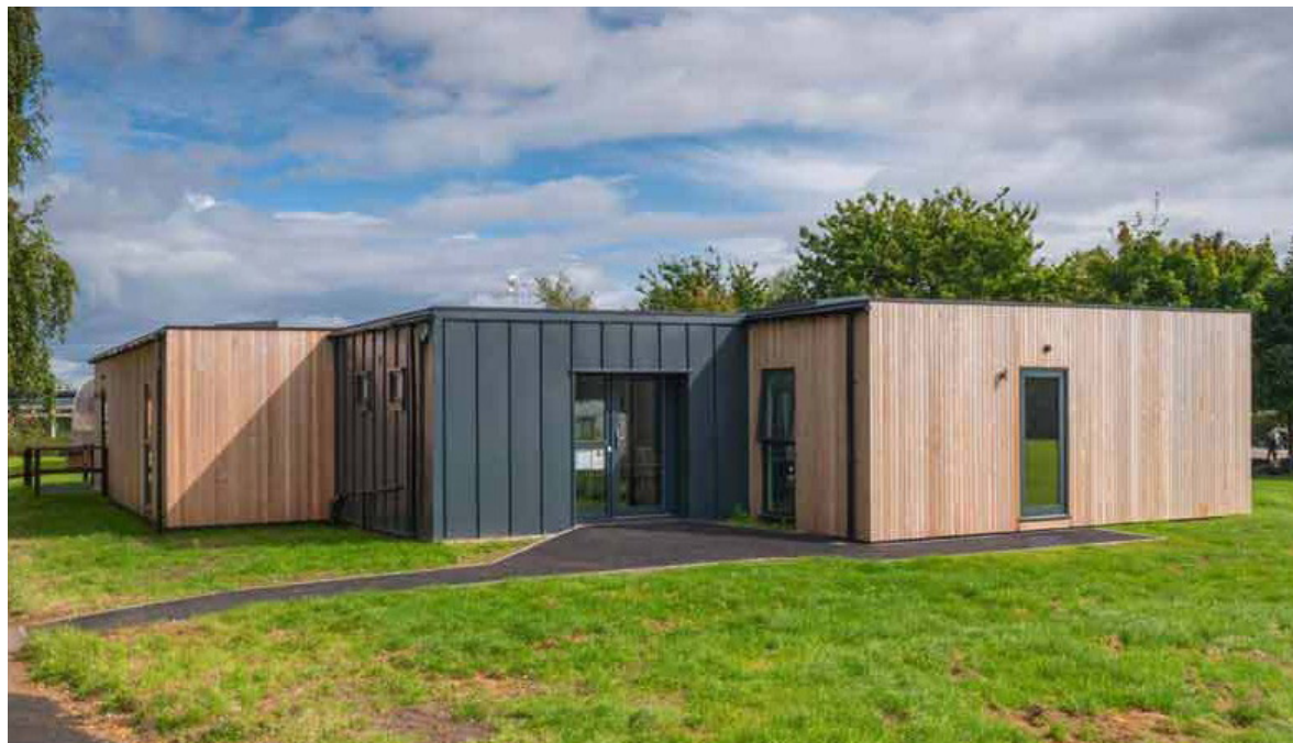
Fig.52 - Vista esterna dell'ampliamento della Sawley Juonior School (Credits: © 2022 Garden Offices da www.greengardenoffices.com/case-studies/full-sized-modular-classrooms-sawley-junior-school-long-eaton )
