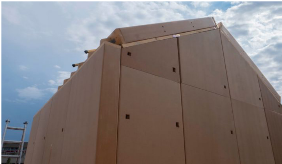
Fig.125 - Sistema a pannelli prefabbricati in cartone PACOTEC™ (Credits: © Archicart®)
