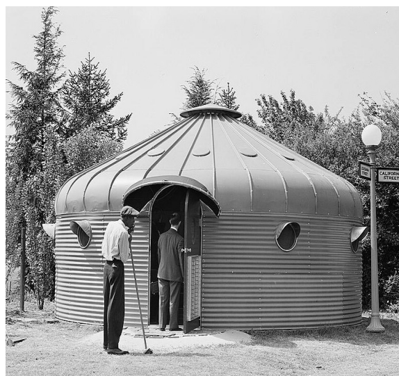
Fig.12 - Dimaxion Deployment Unit (Richard Buckminster Fuller, 1940 ca) (Credits: Foto Daderot da Library of Congress: U.S. Farm Security Administration)
