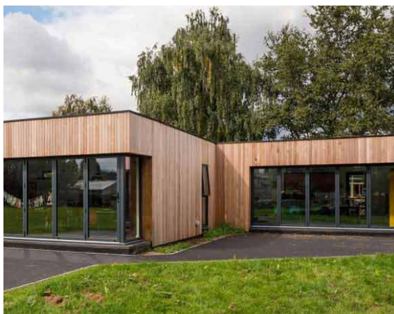
Fig.53 - Vista delle due nuove aule dal cortile della scuola esistente (Credits: © 2022 Garden Offices da www.greengardenoffices.com/case-studies/full-sized-modular-classrooms-sawley-junior-school-long-eaton )
