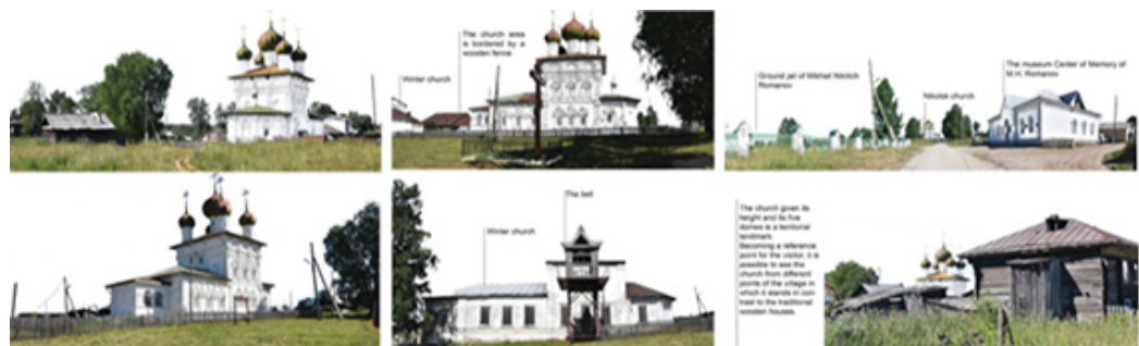
Fig. 5. The relationship between the religious building, still active today, and the territorial context, highlighted in the individual objects that define the complex from the monument and connect to the size of the site. Case study of St. Nikolok church in Nyrob, Cherdyn district.
