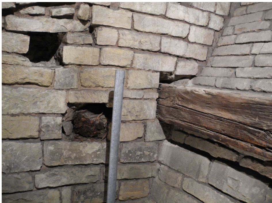
Figure 11. The wooden ties intersect at the corners of the octagonal plan of the Baptistery; the image shows the change in material of the dome at the level of the tie: below the masonry is stone, and above brick.
