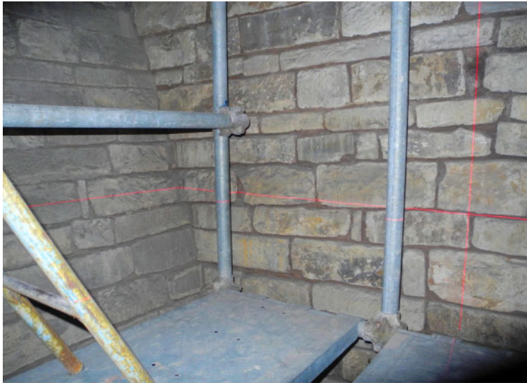
Figure 6. Detail of a partition wall (right) and the extrados of the dome (left) of the Baptistery; the intersection between the vertical and horizontal red lines of the laser highlight the part of the partition wall with masonry in inclined rows perfectly connected with those of the dome.
