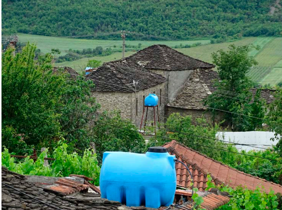
Figure I-4.2.11 Blue water tanks as a hallmark of the urban landscape.
