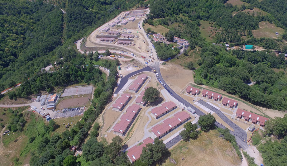
Figure 2. Temporary village of Accumoli case study under construction, 2017.
