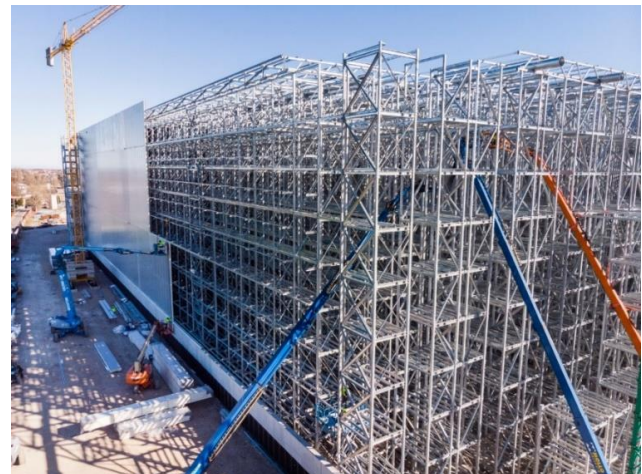
Figure 1 - An ARSW during the construction phase
