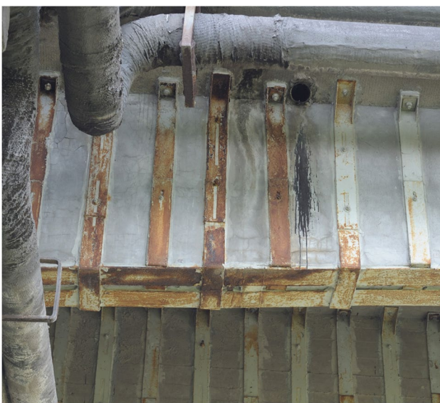
Fig. 10 Longitudinal and transversal bolted steel ties
