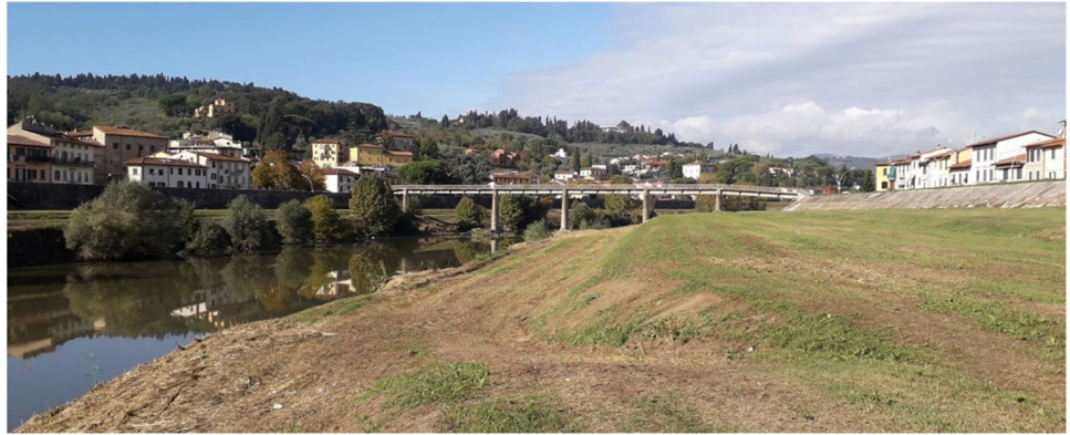
Fig. 5 Walkway, upstream view
