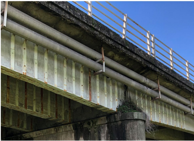
Fig. 9 Ponte sull'Arno, series of bolted steel ties
