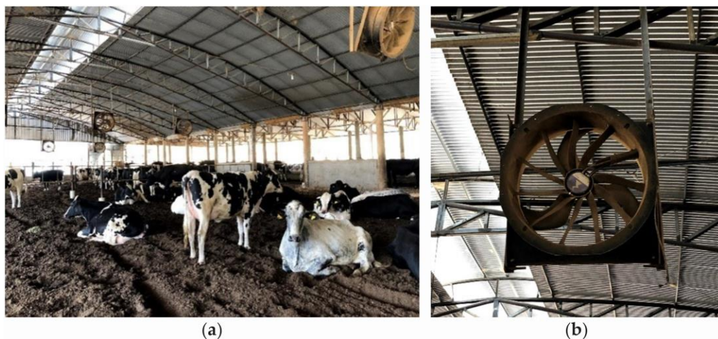
Figure 3. Compost-bedded pack barn system with open sides with automated fans: (a) distribution of fans and (b) detail of the equipment. Source: the authors.
