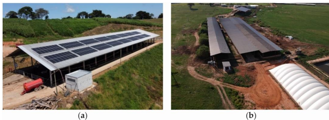
Figure 4. Open compost-bedded pack barn systems with low-volume and high-speed (LVHS) fans and (a) solar panels and (b) biodigesters. Source: the authors.
