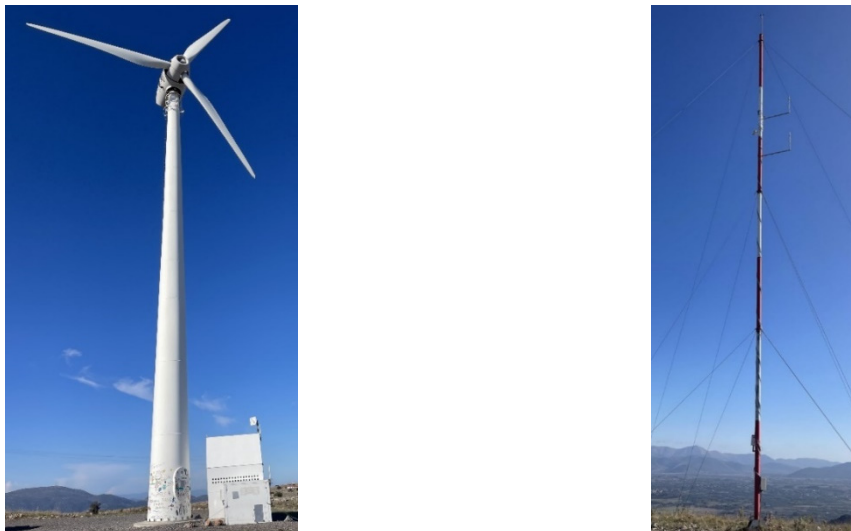
Figure 1: Picture of the Eunice EW16 wind turbine (left) and the meteorological mast (right).
