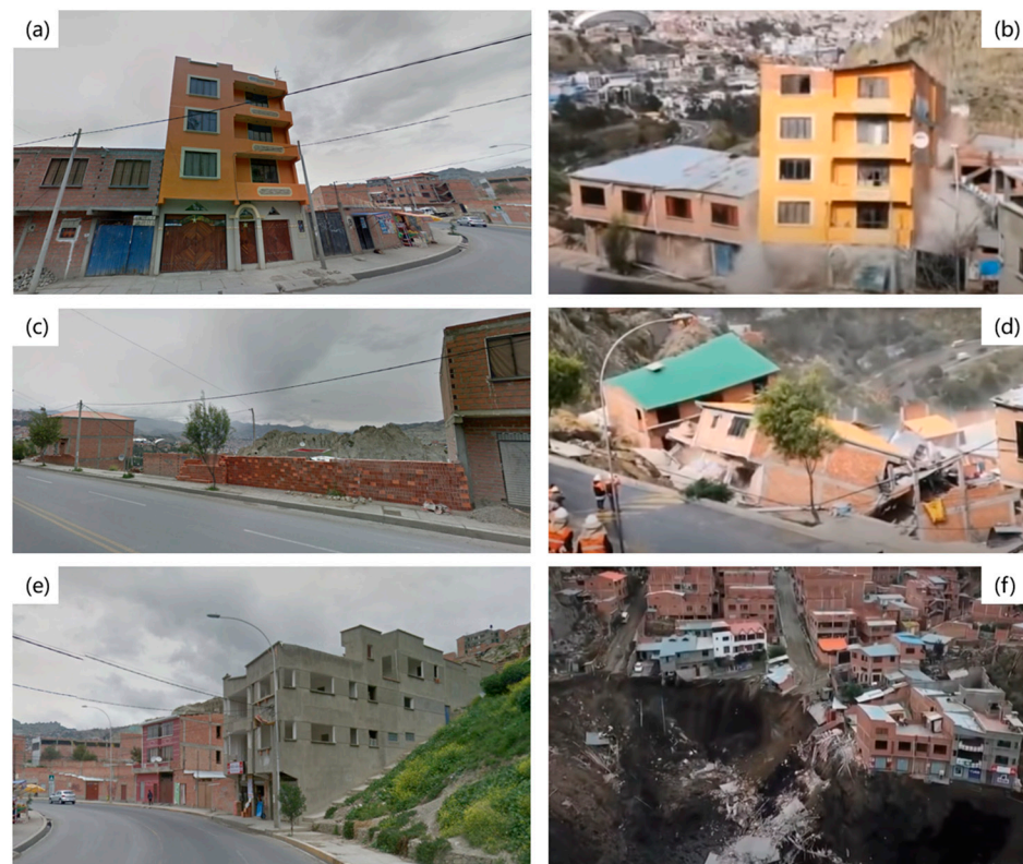
Figure 11. Screenshots taken from Google Maps Street View on the Puente Libertad Road and social media that represent the overload of the landfill caused by the construction work from March 2015 to April 2019. (a) refers to a 3-level building in 2015, and (b) refers to the collapsing building during the landslide. The building had 4 levels in 2019 compared to 3 levels in 2015. (c) refers to a brick wall and according to (d), the former brick wall had been replaced with a building and it collapsed with the two-level building on the left of the picture during the landslide. (e) refers to an unfinished building in 2015 and in (f) the construction had been finished in 2019.
